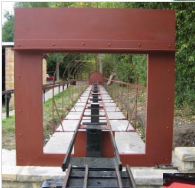
The structure for the second Trolley Shed is progressing well, as these two pictures show. The next stage is to get the doors hung and then clad the structure in the same manner as the first one.
